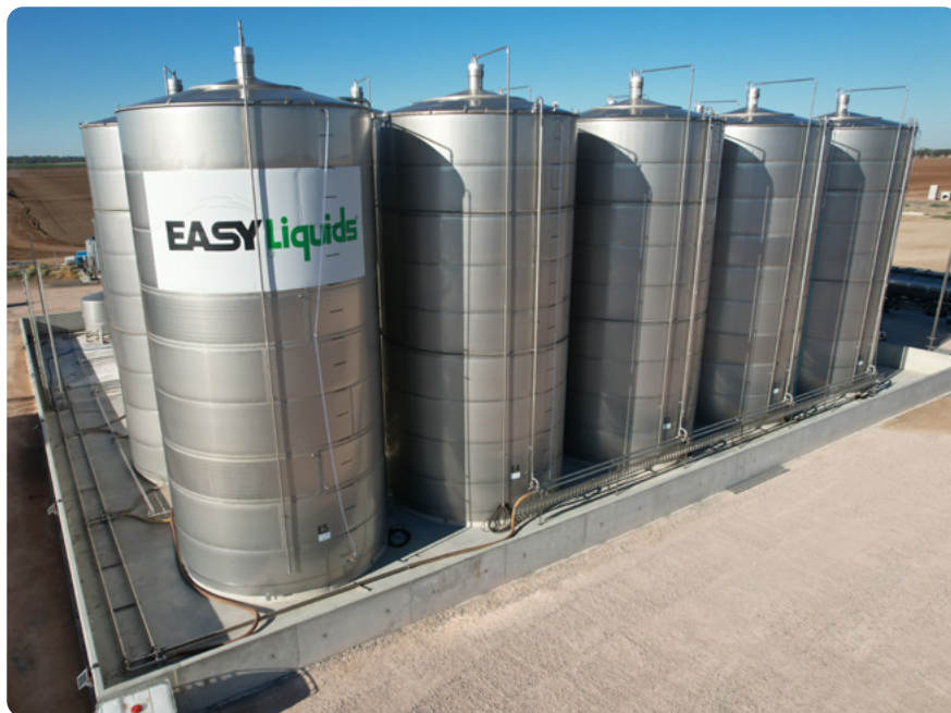
A $2.5-million upgrade of IPF's Whitton EASY Liquids facility was officially opened in February.
