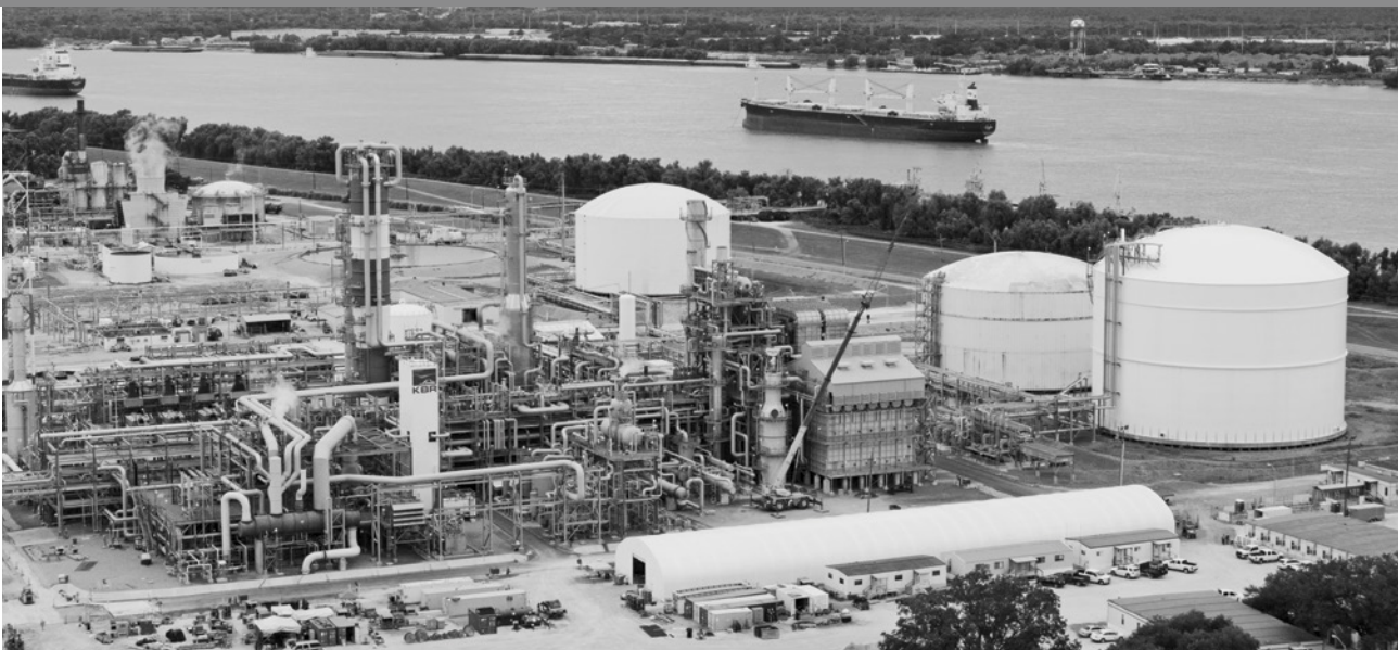
New IPL world scale ammonia plant in Louisiana, USA.
